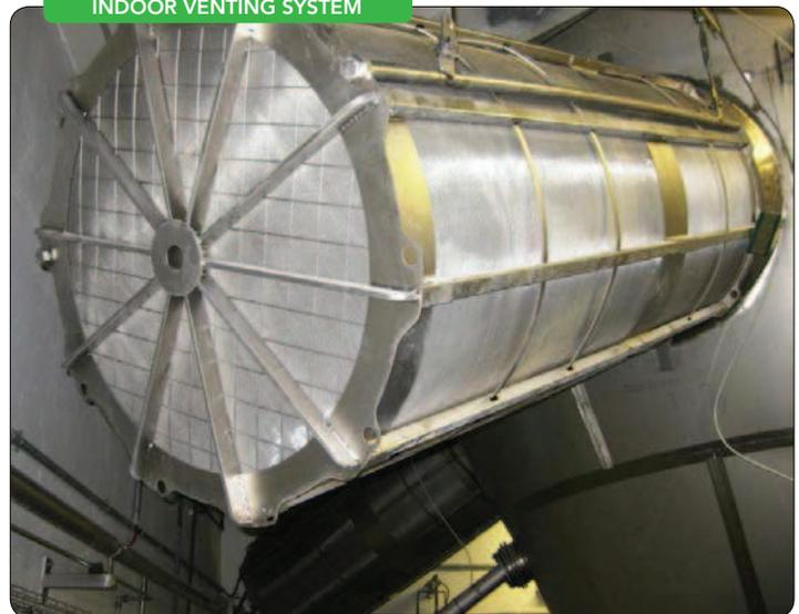
Figure 4. Explosion flame temperatures that reach up to 1,500°C (2,732°F) are efficiently cooled down through an energy transfer taking place in the unique stainless steel mesh filter basket.
